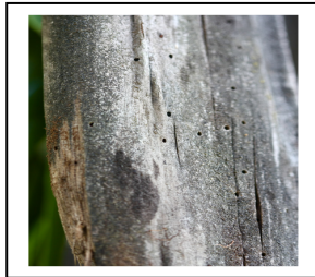
Figure 9: Damage caused by wood borers on tree trunk
